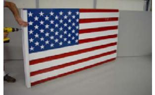
15. Using white screws fasten the trim edge on both ends of the flag. Go through the four prepunched holes into the flag frame. (You will probably want to emove the trim before installation) (see Flag Instillation.)
