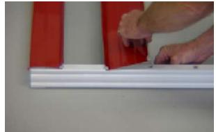
6. All the 5 center red stripes have a lip on both sides that fit under a clip. Take the second red stripe and place one lip under each of the four installed clips. Next insert a clip into the next rafter hole by raising the edge of the stripe so the clip can be placed in the hole. Then lower the edge of the stripe under the clip and snap the other end of the clip into the next hole.
