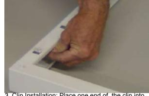
3. Clip Installation: Place one end of the clip into the first square hole coming up from the inside of the rafter. Then push the other end of the clip upward until it snaps into the next hole.
