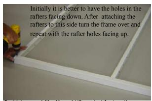
2. Using a drill with a 1/4" socket fasten the rafters to the U channel using the white self drilling screws. Place the screws in the pre punched holes in the U channels. Make sure the rafters are fully inserted into the U channel before fastening.
