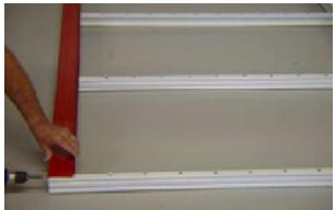
Install the first red stripe: The first and last red stripe have a 90 degree bend on one edge. The other edge has a 45 degree angle and also has a lip on the bottom outter edge that fits under the clip and is secured by the clip. Place this lip under every clip on all four rafters. Using the red screws fasten the first red stripe at the four prepunched holes.
