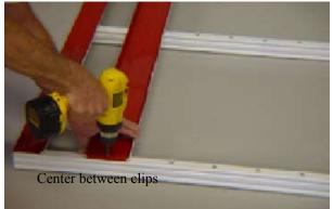
7. After the 2nd red stripe is secured by four clips fasten the stripe at both ends using a red screw. The ends of the stripe must be just inside the outter edge of the of the two outside rafters. Also center the stripe between the clips on the outter fafters. There are no pre-punched holes on the ends of the stripes. The self drilling screws will drill its own hole.
