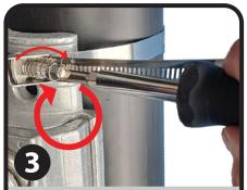
Press the tension screw against the Strap and tighten it by turning the screw. Attach a Mounting Strap onto the Bracket flange's lower mounting channel, attach a 2nd Strap to the upper Bracket flange. Tighten all Strap screws.
