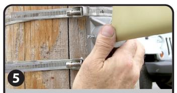
Insert the clevis pins through the open hole. Note: A mallet or hammer may be necessary to tap the pins through each of the holes.
