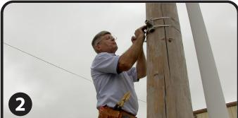
Set the top bracket (with the arrow pointing up) to the desired height on the pole. Secure the bracket in place with two release bands.
