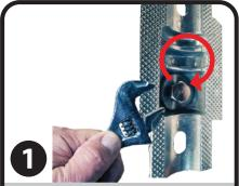
Before beginning the install, turn each Spring Loaded Bracket around and tighten the 3/4" bolt head that is located on the back.
