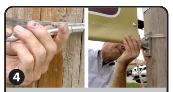
Set the bottom bracket (with the arrow pointing down) to the desired height on the pole. Secure the bracket in place with two release bands.
